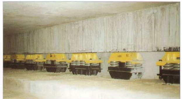
Spring elements in final position
