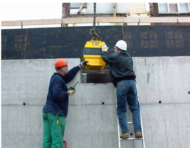
Placing of a spring element
