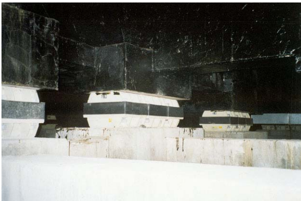
Spring system in operation
