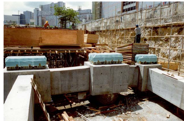
Spring elements placed on pile caps
