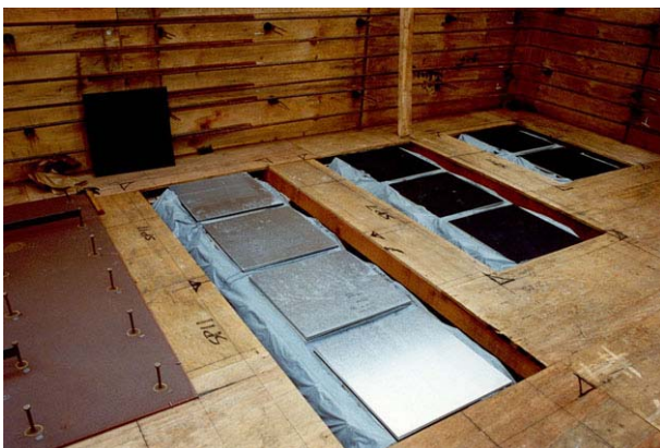
Spring elements embedded in soffit formwork
